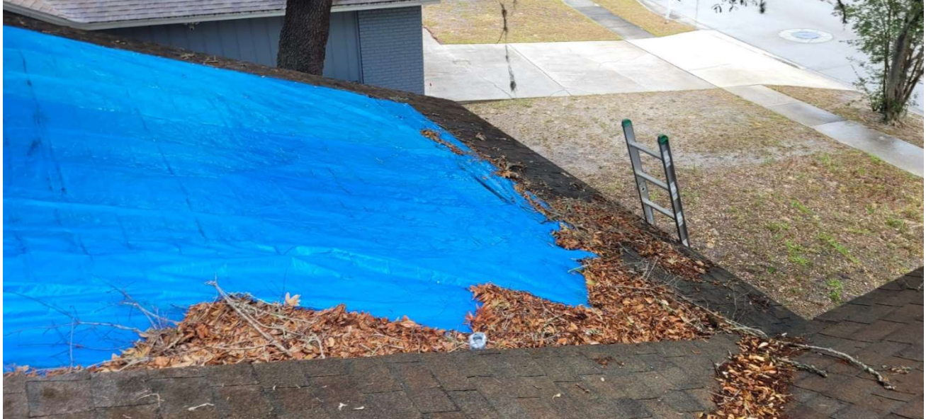
Exiting tarps (2) from prior contractor
